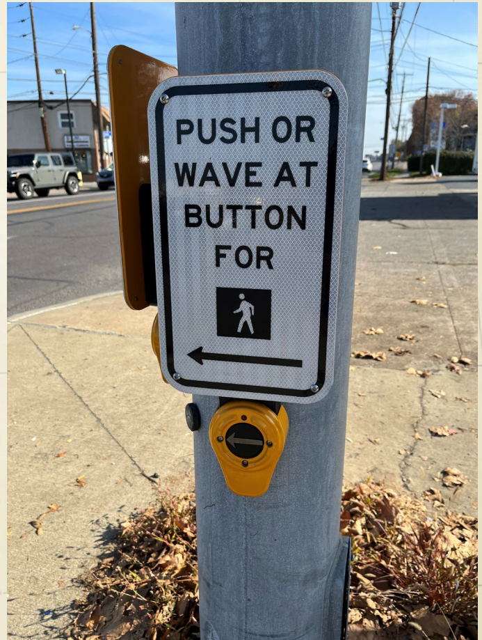
Accessible Pedestrian Signal Example
