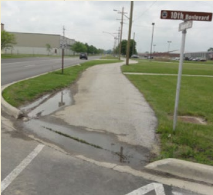
Curb Ramp with Ponding
